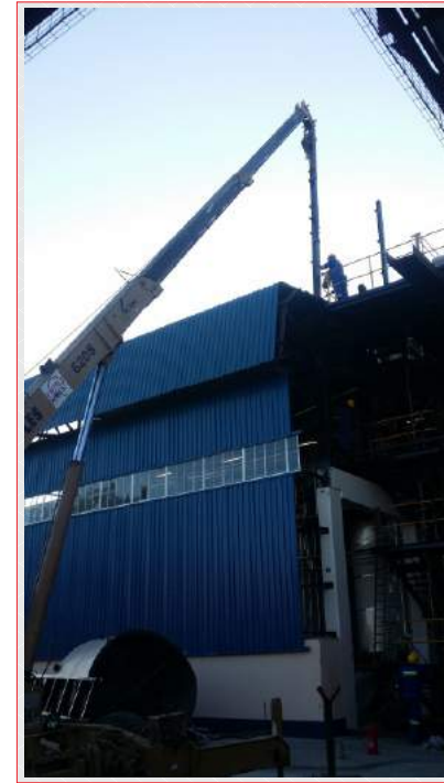
Erection of Mono Pitch High Roof.
