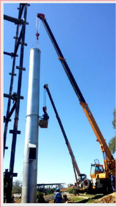
Installation of 31m High Chimney Stack
