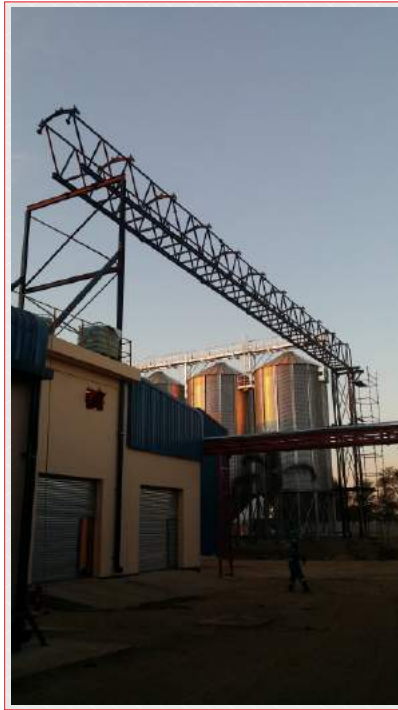
Service & Walkway Bridge Fabricated & Erected.
