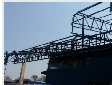
Fabrication & Erection of Canopy Steelwork
