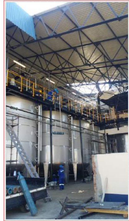
Erection of New Stainless Steel Tanks
