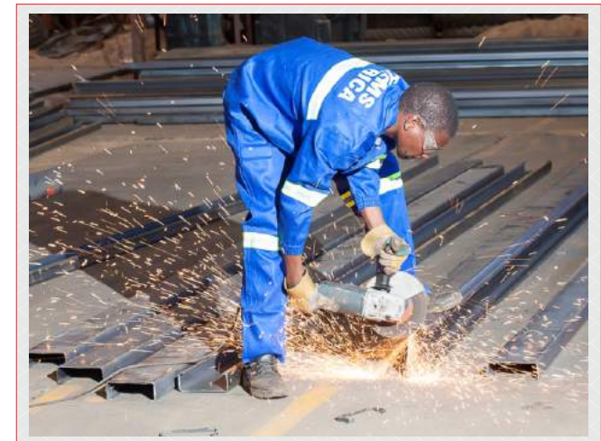
Steel Fabrication & Welding
