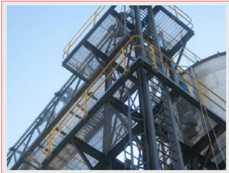
Service Bridge Tower Installing handrailing & Open Grid Flooring.
