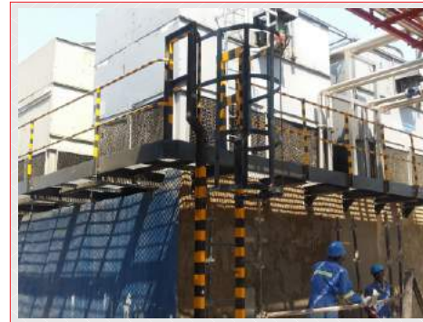
Water Cooling Plant Erected.
