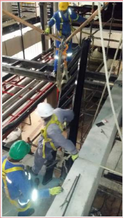
Rigging in Constricted Areas
